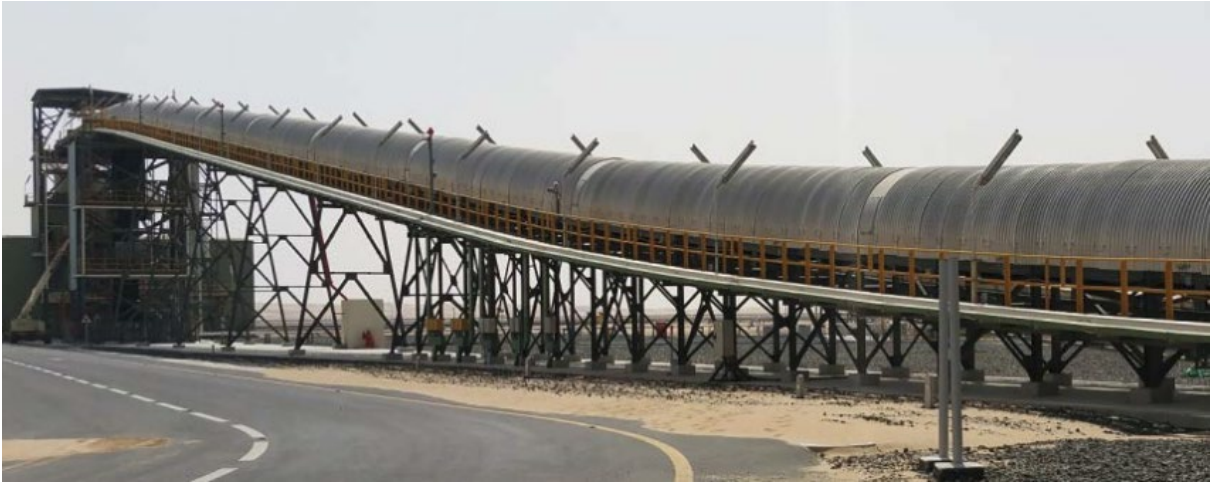
Photo 2: Reference Belt Conveyor and Transfer Tower
