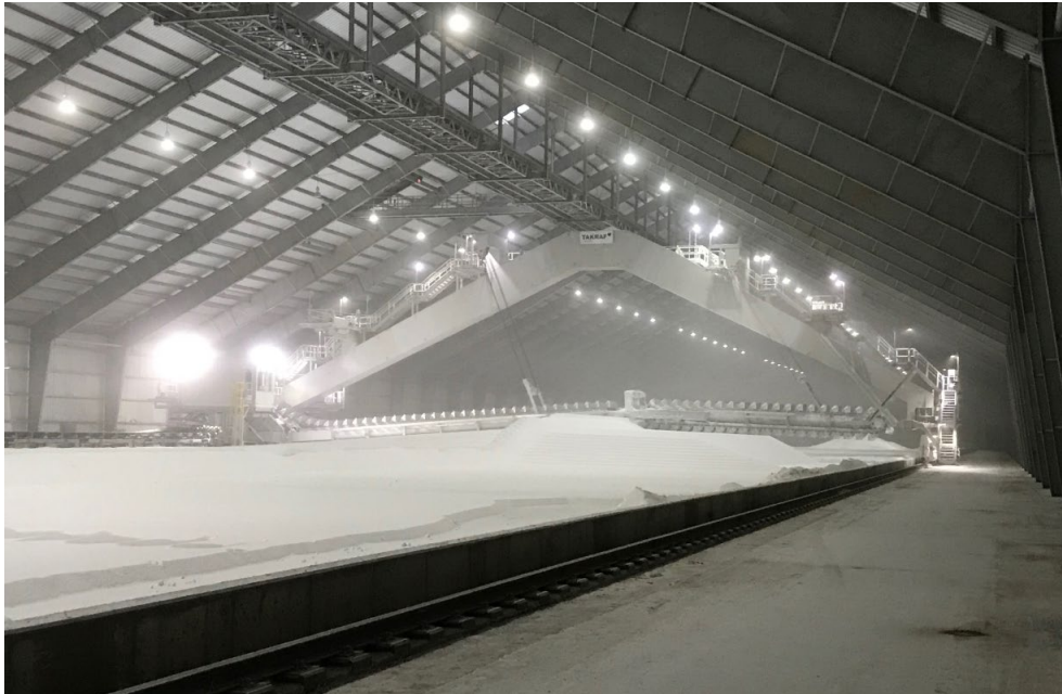
Photo 3 : Urea Storage Building
