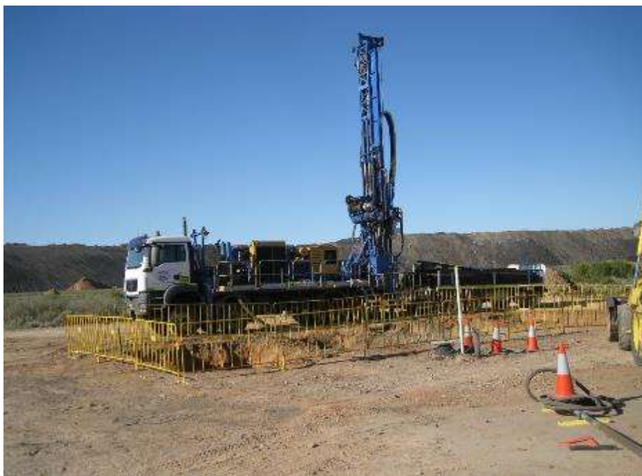
Figure 3-1: Typical layout of an exploration drill site
