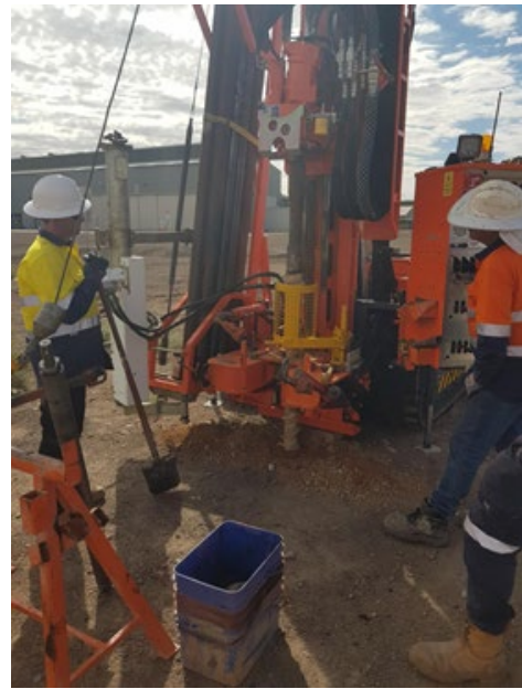
Drill rigs and teams geotechnical investigations associated with the construction of the NRUP) gasification wells and power generator areas.
