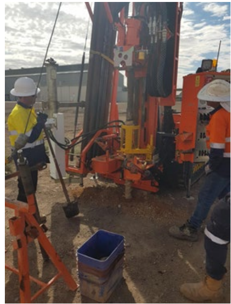
Drill rigs and teams geotechnical investigations associated with the construction of the NRUP) gasification wells and power generator areas.
